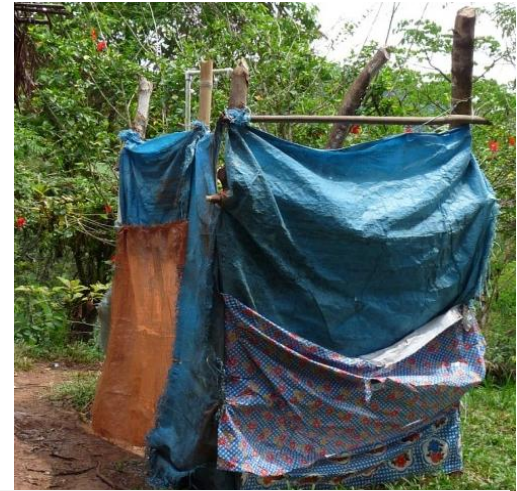
Pit Latrine in Oma, Panama. Example of superstructure with limited security, privacy, or shield from weather.
