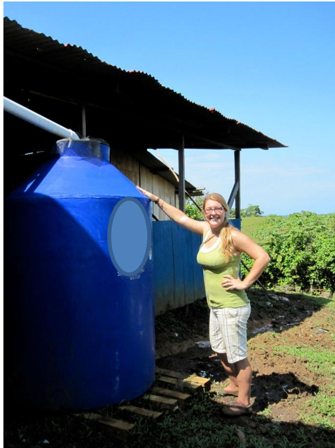
Figure 3: A Rainwater Harvesting System Made of the Plastic Tank Option
