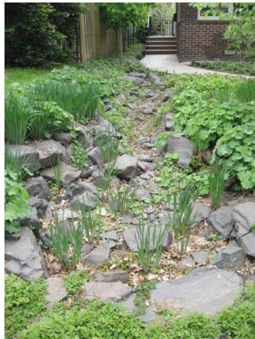
Figure 2 – Bioswale, Minneapolis, MN (Putnam, 2010)
